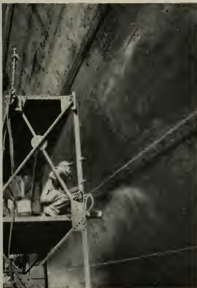
▼ Below: Shipping Copper being applied to Pope & Talbot's Laura Bridgeman.
